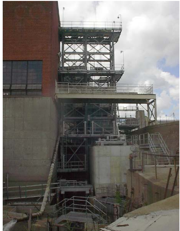
FIGURE 5 LOOKING UPSTREAM AT THE FISHWAY AFTER RENOVATION IN 2004
