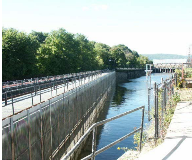
FIGURE 7 LOUVER ARRAY IN FIRST LEVEL CANAL
