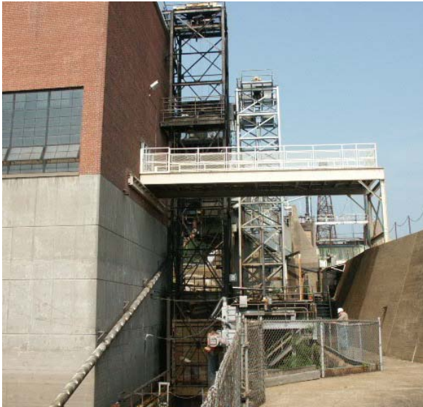
FIGURE 4 LOOKING UPSTREAM AT THE FISHWAY PRIOR TO RENOVATION IN 2004
