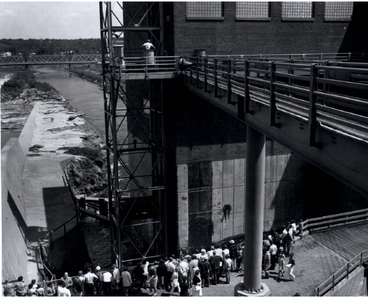
FIGURE 2 LOOKING DOWNSTREAM AT THE FISHLIFT
