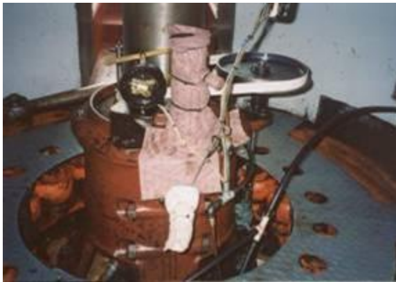
PHOTO 8 ORIGINAL TURBINE GUIDE BEARING INSTALLATION
