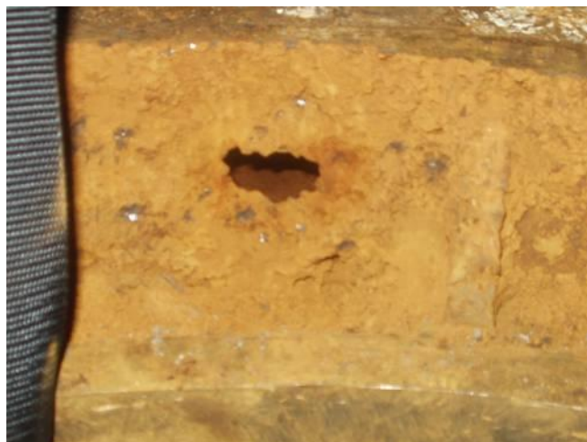
PHOTO 4 DISCHARGE RING CONDITION
