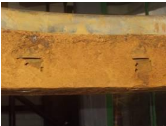
PHOTO 6 EXPOSED WICKET GATE BUSHINGS
