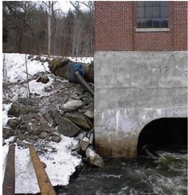
PHOTO 10 TURBINE BYPASS
