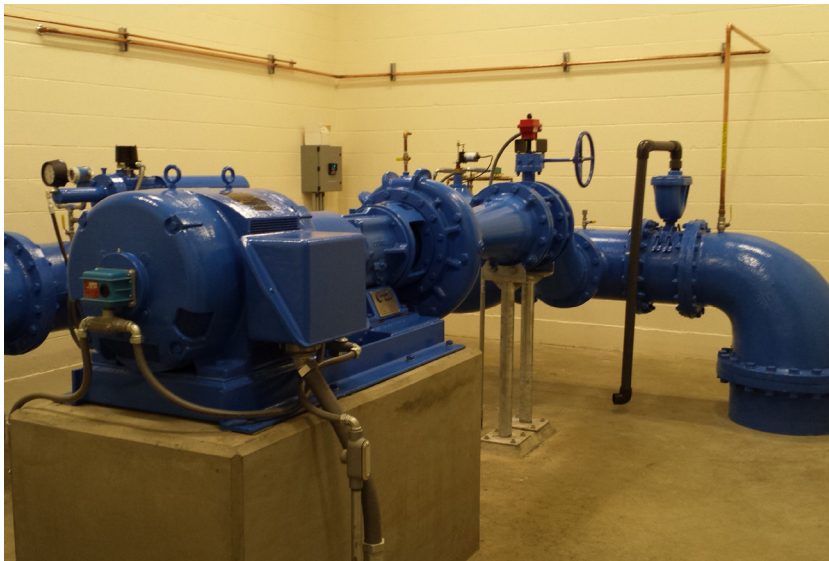
This is an example of a pump-as-turbine unit. Photo courtesy of Canyon Hydro
